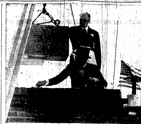
Grand Master Walter Raacke, assisted by grand marshal, laying corner-stone of student-faculty building at Wayne State Teachers College. Photo by John A. Moore
